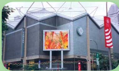
VHB tape was used to bond the wall cladding of Suntec City Building.
