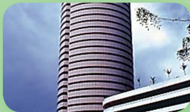
VHB Tape was used to bond flat corrugated aluminum stiffener sections to curtain wall panels in this 55-storeys Singapore Temasek Tower.
